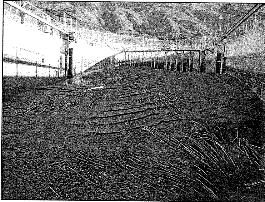
Photo 13- Sediment inundation in Robles Diversion screenbay prior to emergency cleanout
